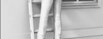
FIG. 1 CORRECT - USER MAINTAINING THREE POINTS OF CONTACT (MEANS OF SECURING OMITTED FOR CLARITY)
